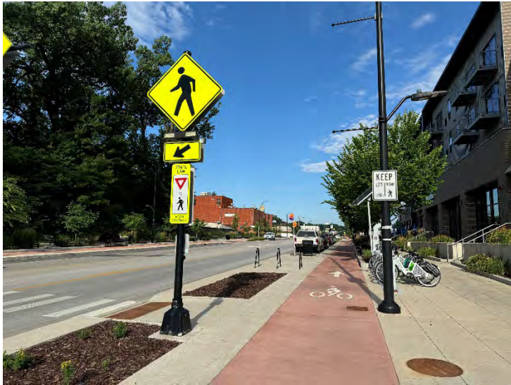
Figure 80: Example Curb-Separated Bike Lanes
