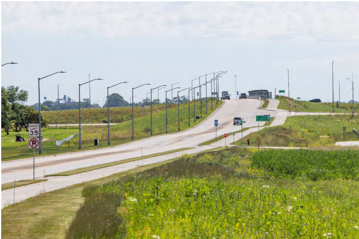
20 th Street South Interchange (I-29 Exit 130)
